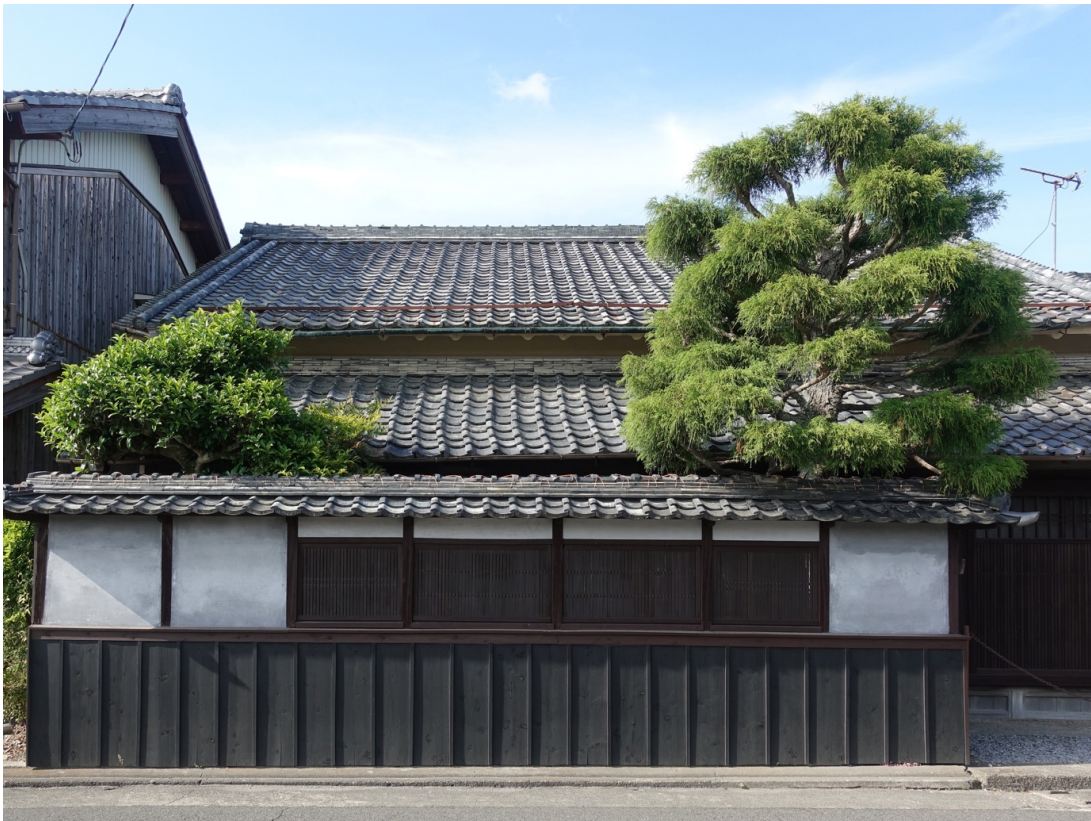
Figure 5. Restored wall of Nishida Residence (19 May 2019 by Arno Suzuki)
